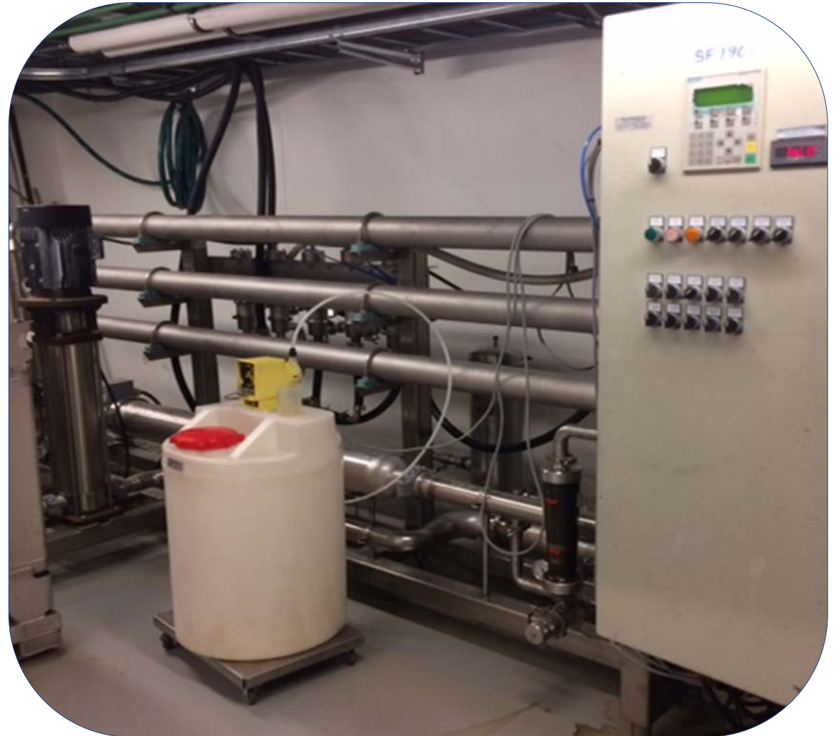
DEMO SCALE NF PLANT OF 98 m 2 FILTRATION AREA FITTED WITH GE HL MEMBRANE
