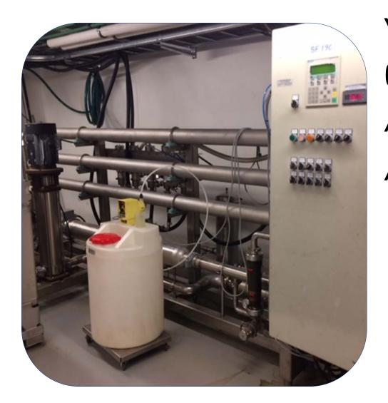
**VOLUME CONCENTRATION FACTOR** (VCF) = FEED VOLUME/CONC.VOLUME AVERAGE RETENTION=(1-C<sub>P</sub>/C<sub>AV</sub>)\*100% AVERAGE FLUX=  $V_P/(A*T)$
